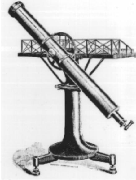
FIGURE 1. Sketch of the Almucantar used by Chandler to detect polar motion.
