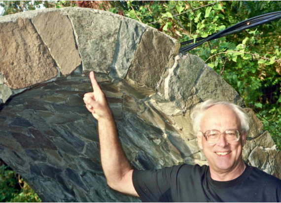
Bob pointing to the keystone in a stone arch (Photo by Robert Steneck.)
